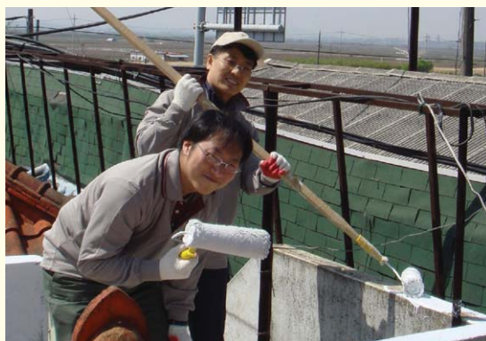
• Repair Work at New Heaven Shelter
